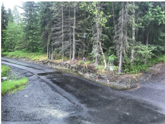
Figure 2 Cut and fill w/ unfinished shoulders
