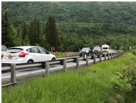
Figure 12 Common traffic congestion in proximity of Kenai River Bridge
